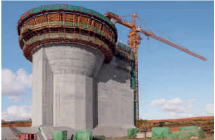
Freeform formwork on SCS Climbing Brackets for a large-sized concrete funnel.
