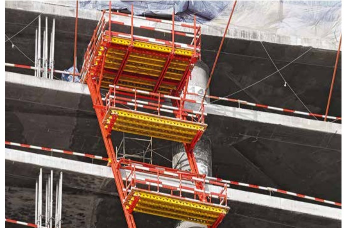
Landing Platforms can also be rail-climbed by means of the mobile RCS Climbing Hydraulics – this additionally minimizes crane usage.
