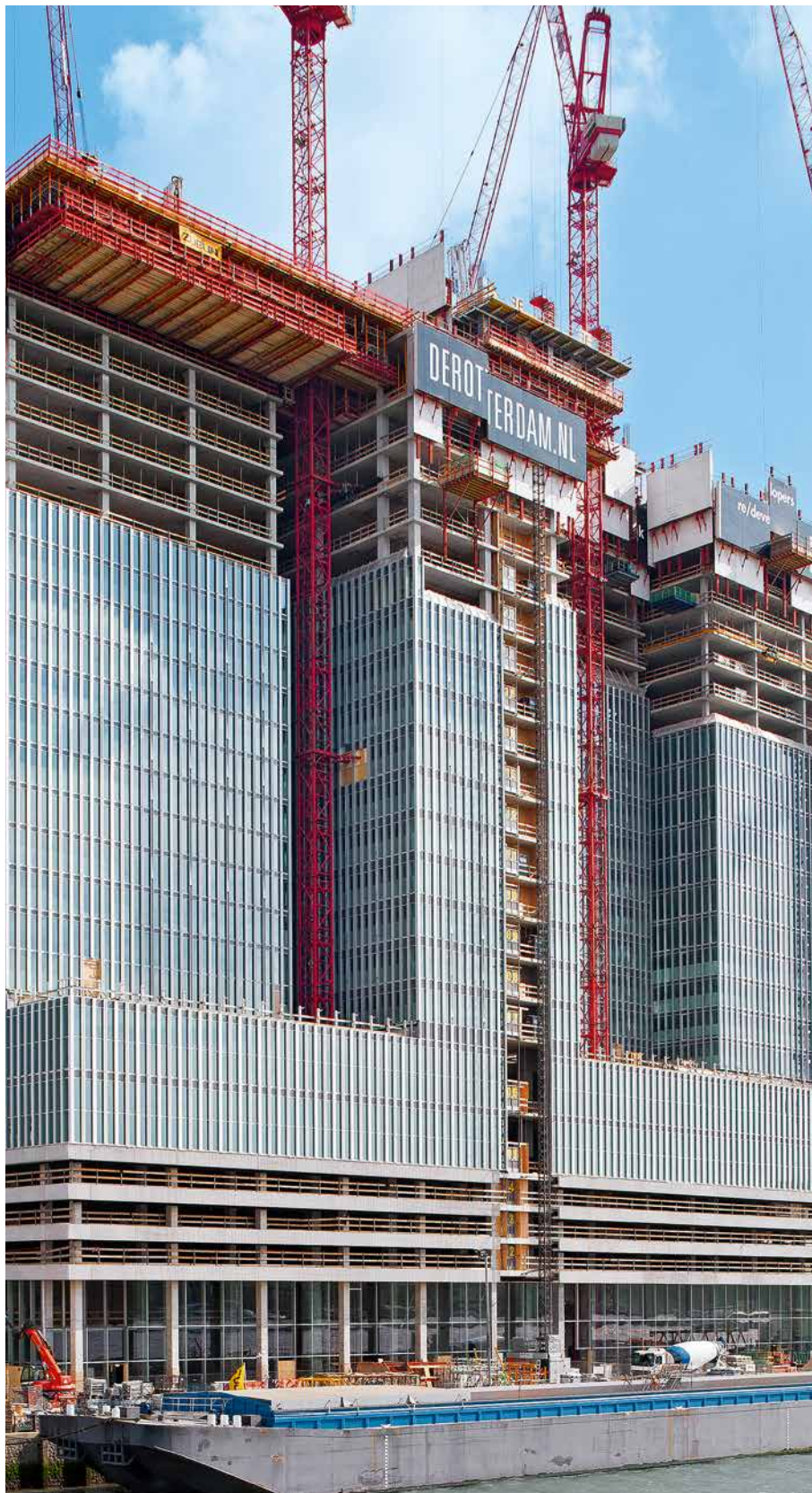
De Rotterdam, Rotterdam, Netherlands Complete enclosure with the RCS P Climbing Protection Panel provided maximum protection and facilitated a safe and fast working environment in the two topmost floors under construction. An important element of the PERI solution was the VARIOKIT truss construction for supporting the up to 9 m cantilevered floors at the halfway point of the building.
