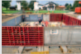
Wall Formwork
