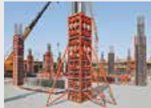
Column Formwork
